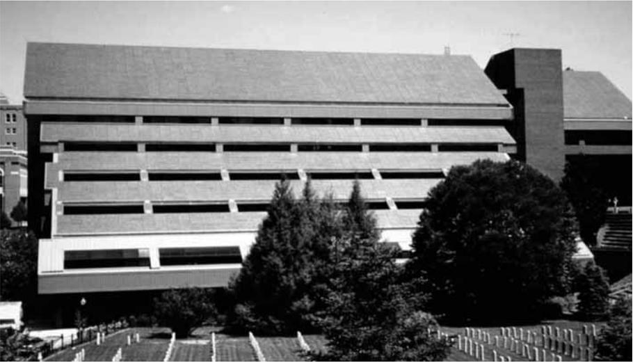
**Figure 4.1** *Roof-integrated Photovoltaic System [Georgetown University in Washington (USA), Installed in 1984 with 4464 Photovoltaic Modules and 337 kW<sub>p</sub> Total Power]*
